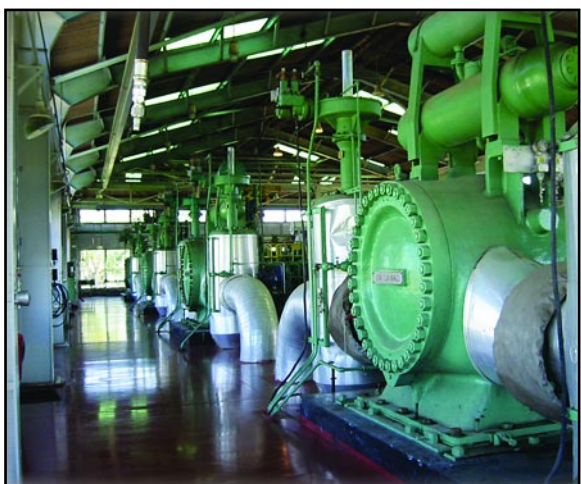
Figure 4. Centrifugal compressor
