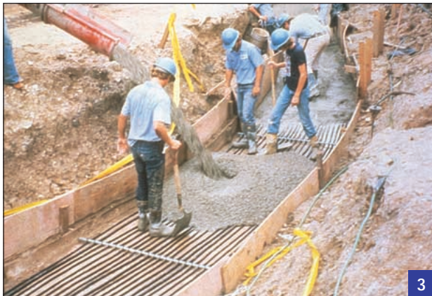
Underground direct buried system.
