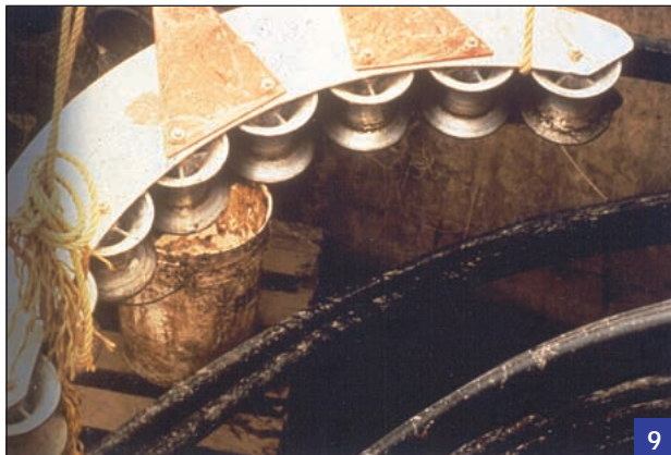
Use of rollers to minimize bend damage.
