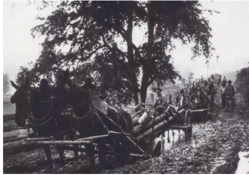
Figure 5. Stringing wagons haul pipe to the right-of-way, circa. 1900. Photo courtesy of East Ohio Gas Company.
