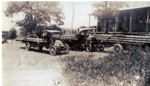
Figure 6. Stringing wagons have been replaced by trucks, but their purpose is the same, circa. 1924. Photo courtesy of Maurice Yost family archives.
